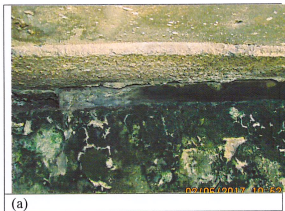
Figura 41: (a) ressecamento do neoprene
